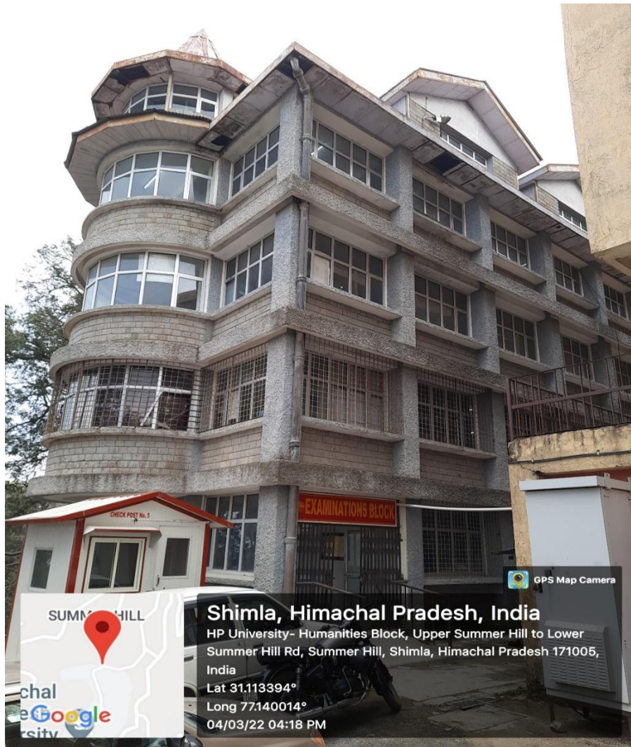
Examination Block Building
