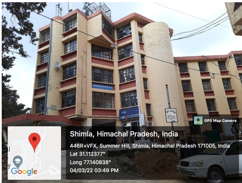
Administrative Block Building
